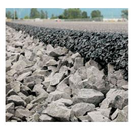
Porous asphalt pavement can filter stormwater and mitigate runoff effects. (Image courtesy of Century West Engineering)
