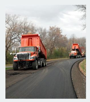
Northeast Asphalt repayed Calumet County Park's roads with rubber-modified asphalt. (Image courtesy of Northeast Asphalt)
