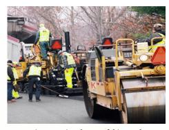
NAPA is promoting the use of thin overlays to extend the life of asphalt pavements. Thinlays protect pavements, restore ride and improve safety and structural capacity. (Image courtesy of NAPA)
