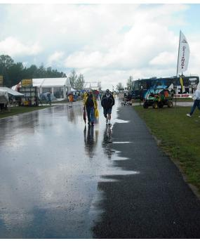
Strategically placed porous pavement at Wittman Airport in Oshkosh handles the stormwater runoff for the entire pavement. (Image courtesy of OMNNI Associates)
