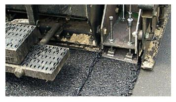
The notched wedge joint prevents the slope of a joint from tapering to thin, low-density material. (Image courtesy of the Asphalt Institute)
