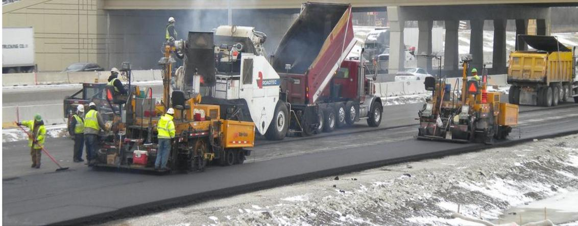
**Failing densities with PG64-22 HMA.**
