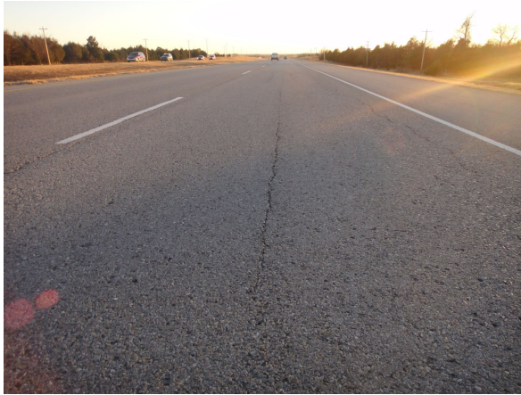
Longitudinal Cracking (Not in Wheelpath)
