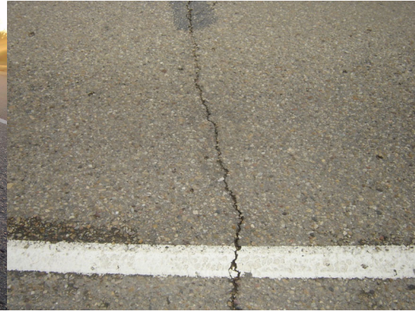
Low-severity thermal cracking
