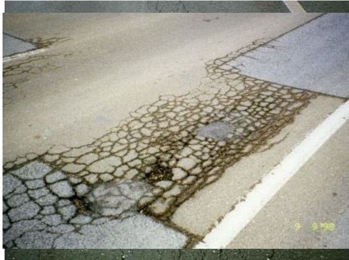
Fatigue cracking
