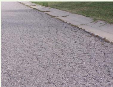
Figure 4 This pavement remains incomplete. The surface layer was never built, even after all of the subdivision lots were developed.
