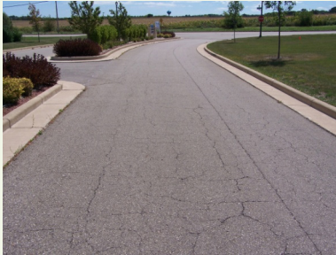
Figure 3 A binder layer showing fatigue distress, which results from a first-stage pavement structure that is underdesigned for the loading conditions
