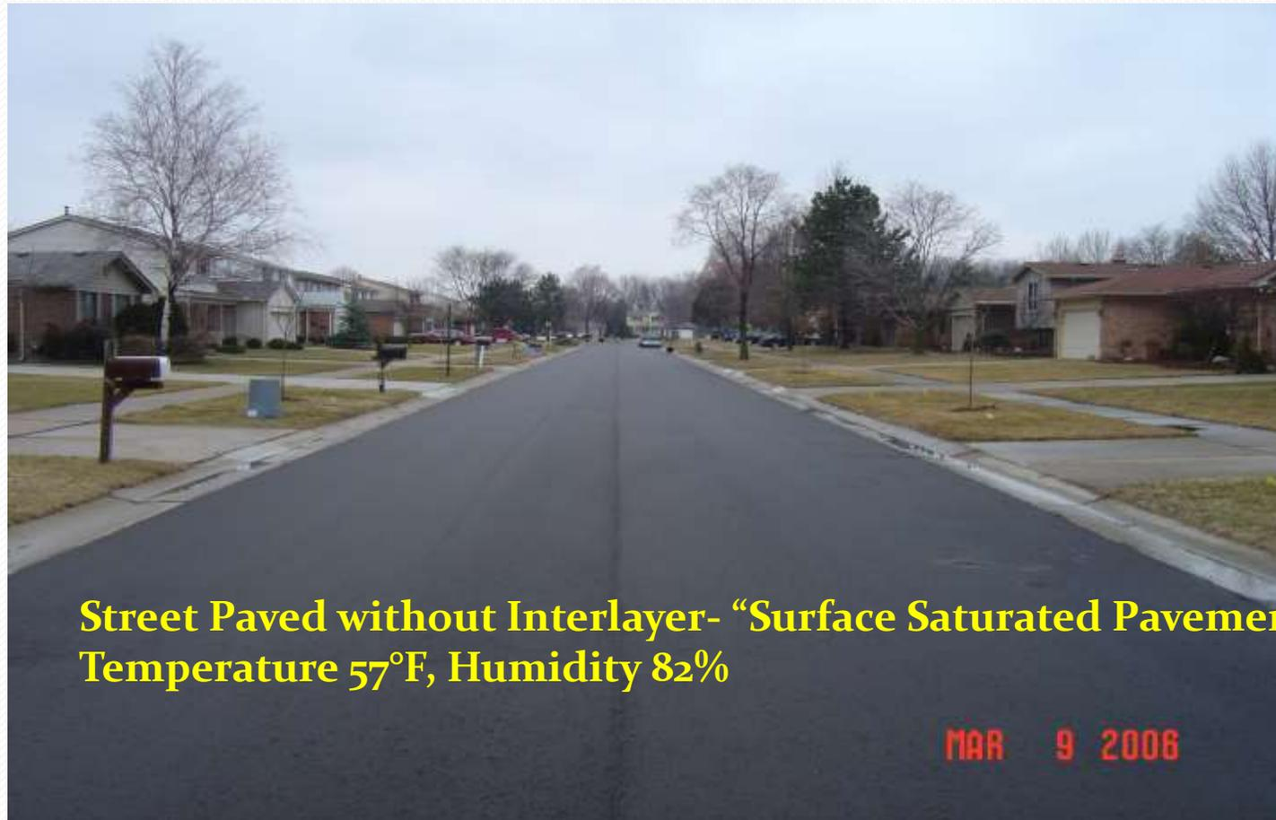
**Street Paved without Interlayer- "Surface Saturated Pavement"**
