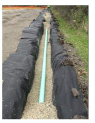
Figure 7. An image of a French drain.<sup>6</sup>
