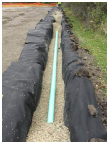
Figure 7. An image of a French drain.<sup>6</sup>
