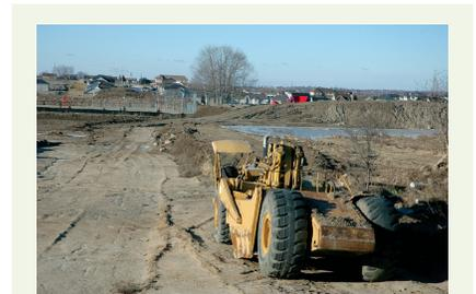
**Figure 2** The quality of the sub-grade soil plays an important role in determining pavement thickness.
