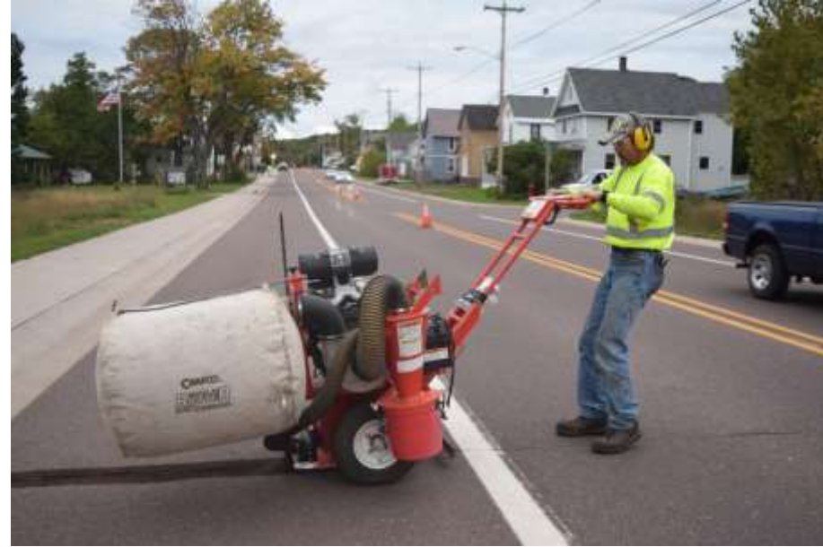
Photo Above: New OSHA Required Routing, Effective Dust Suppression System
