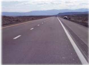
PG 64-22 modified, no rutting
