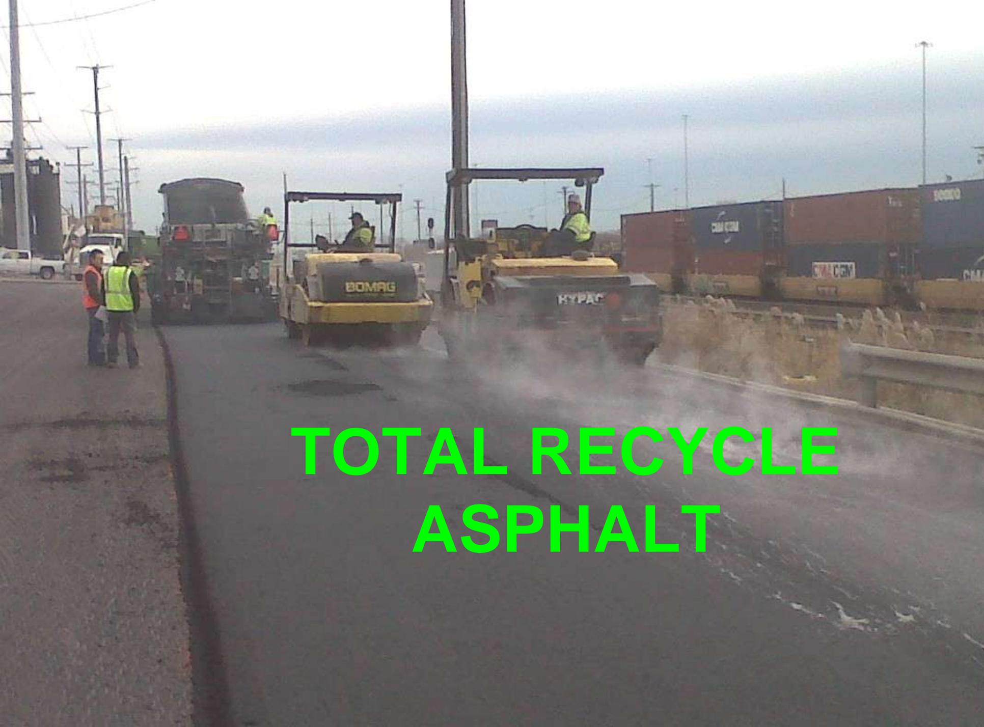
A construction site showing the paving of a road using Total Recycle Asphalt. In the foreground, a yellow BOMAG roller is followed by a larger yellow HYPAC roller, both emitting steam or dust. To the left, two workers in high-visibility vests stand near a large truck. In the background, there are utility poles, a white car, and a train with blue and red containers. The sky is overcast.
