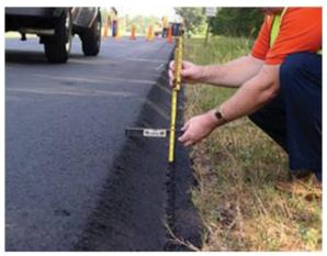
Figure 6.2. Safety Edge (Image courtesy of WisDOT)
