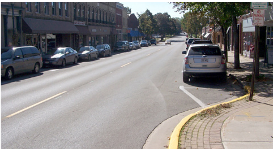
Three years later, downtown Ripon's asphalt replacement keeps delivering trouble-free performance.
