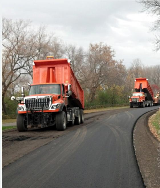
*Northeast Asphalt repaved Calumet County Park’s roads with rubber-modified asphalt. (Image courtesy of Northeast Asphalt)*
