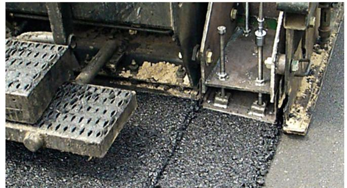
The notched wedge joint prevents the slope of a joint from tapering to thin, low-density material. (Image courtesy of the Asphalt Institute)
