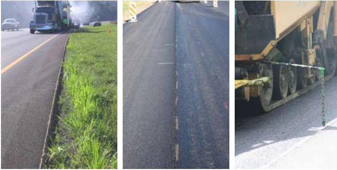
Stringline for reference, and/or Skip Paint, Guide for following
