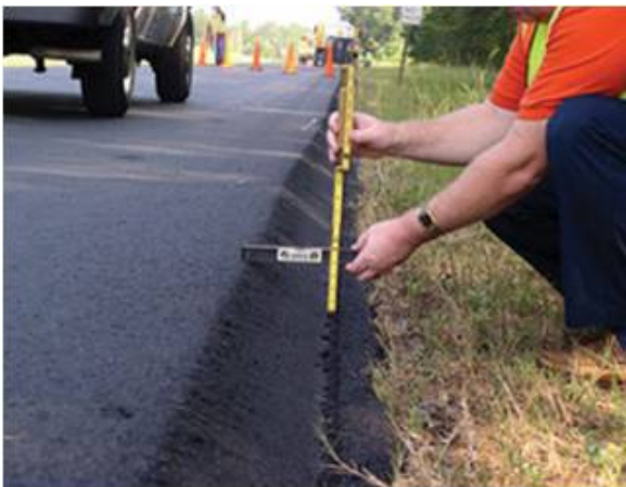
Figure 6.2. Safety Edge (Image courtesy of WisDOT)
